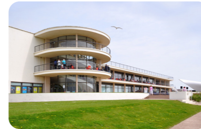
De La Warr Pavilion, England
